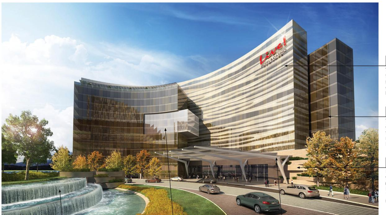
The Main Hotel Tower façade features undulating and sinuous horizontal patterns on dark brown glass created by high quality ceramic fritting.
