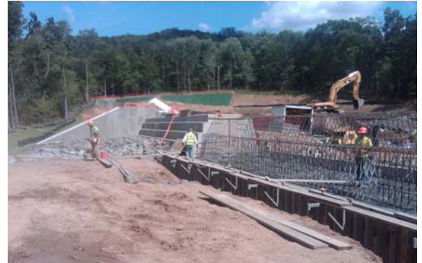
New Dam and Detention Basin Under Construction
