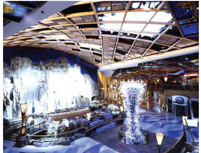
Barrel Vault Ceiling
