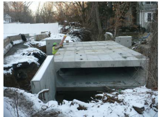
Drainage-Phase II Schuyler Road Box Culvert Installed
