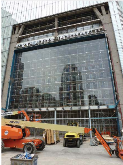
World Trade Center South Curtain Wall
