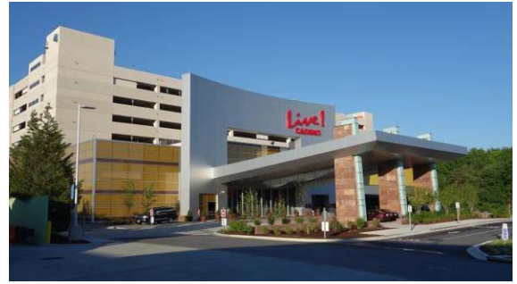
North Elevation of Maryland Live
