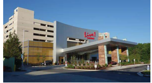
North Elevation of Maryland Live!
