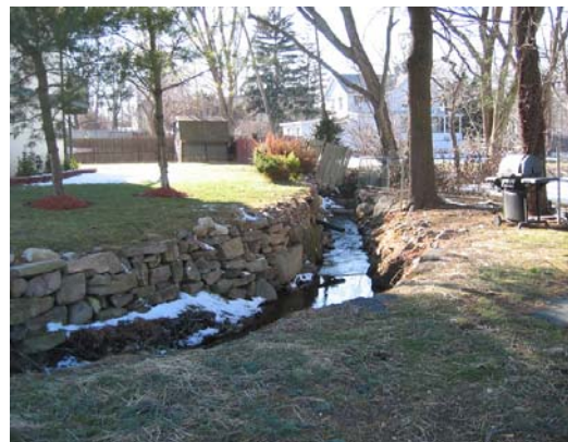
Detention Basin with High Berm (Before)
