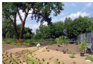
Bioswale Under Construction
