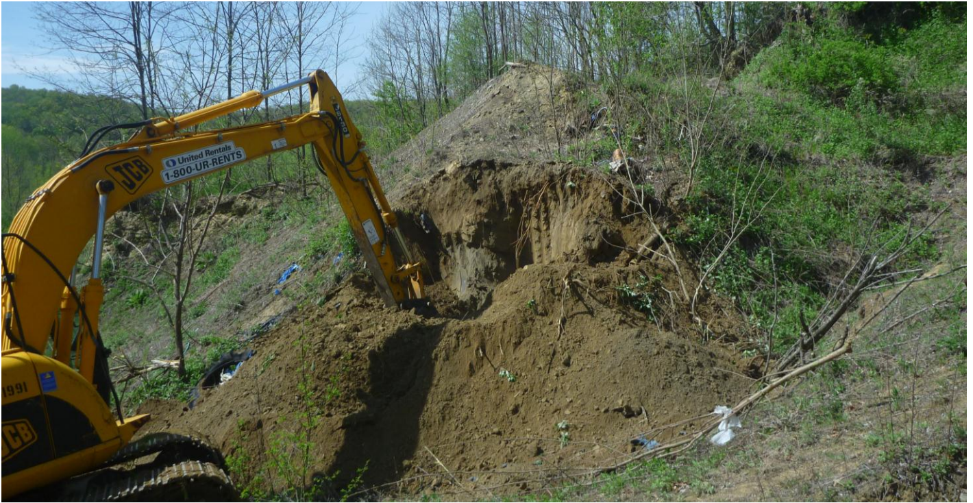
Photograph 13: View of the clean sand observed at TP-9
