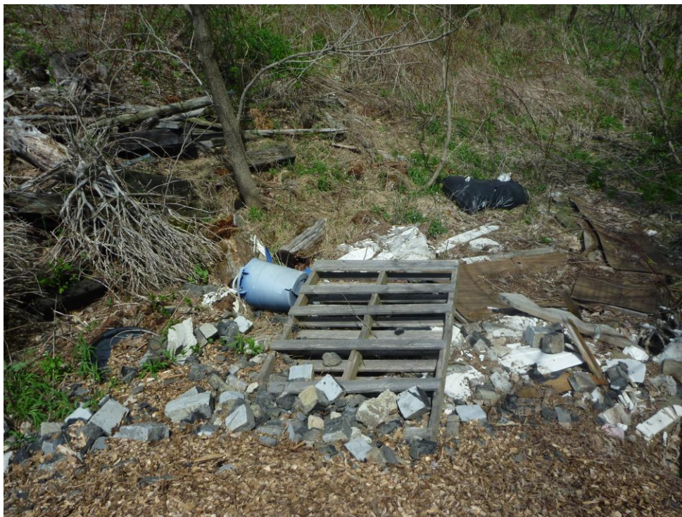
Photograph 19: View of Debris Pile #9 (Parcel #1), containing roofing waste, tires, concrete chunks, etc. View from north to south.
