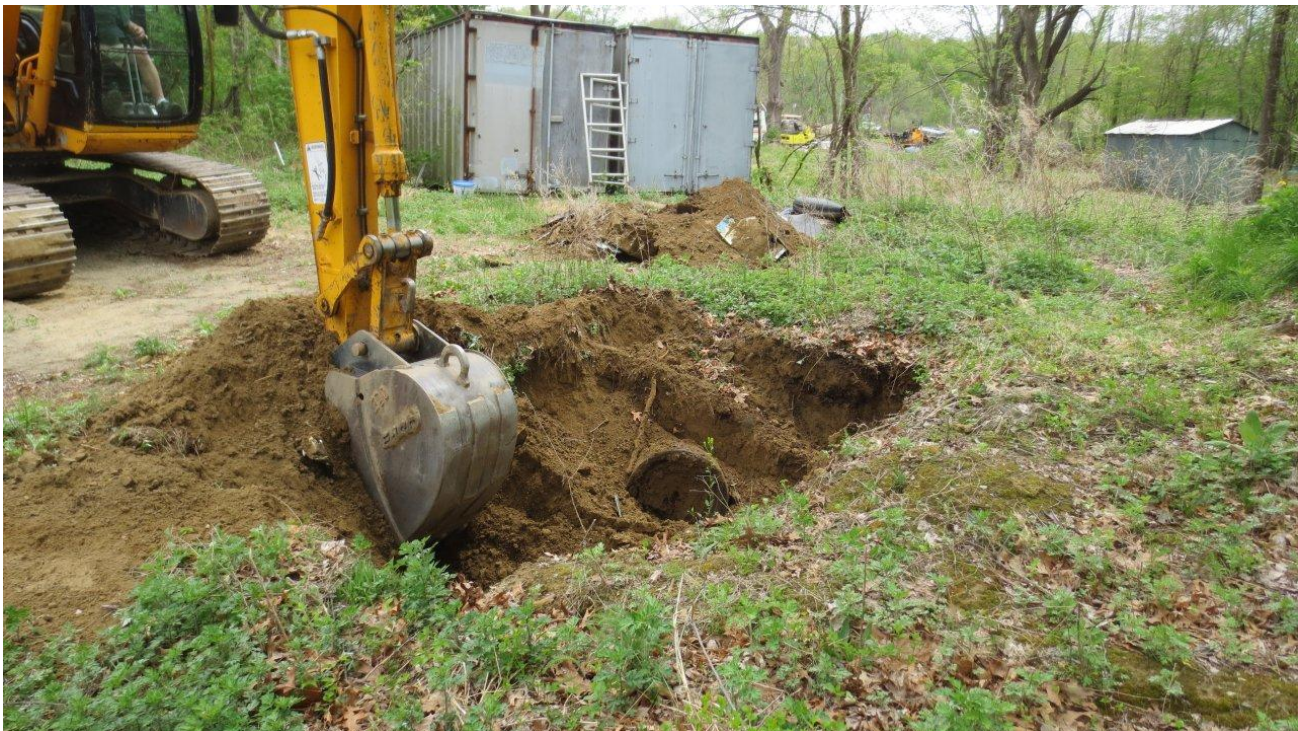
Photograph 8: View of the excavation of TP-7, facing east.
