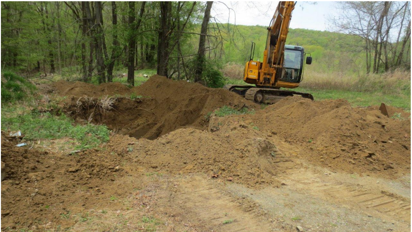
Photograph 9: View of the material excavated from TP-7, facing west.
