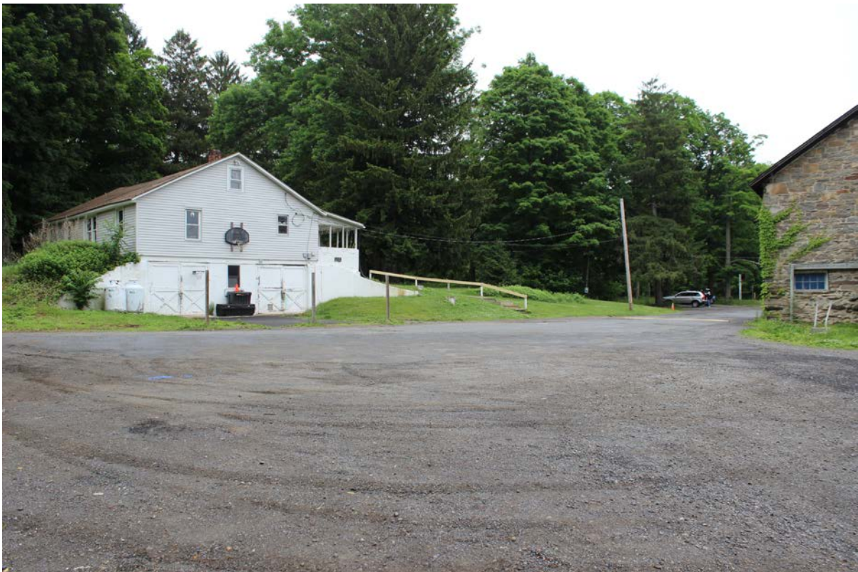
Photo 4 – Existing Residential Structure
