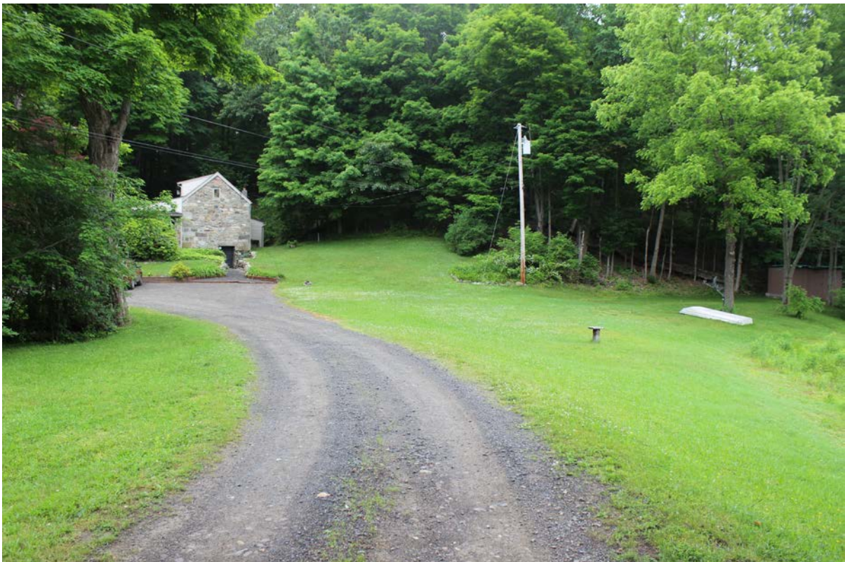
Photo 8 – Existing Residential Structure, near pond
