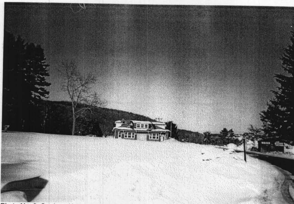
Photo No. 3: Carriage House, under renovation.
