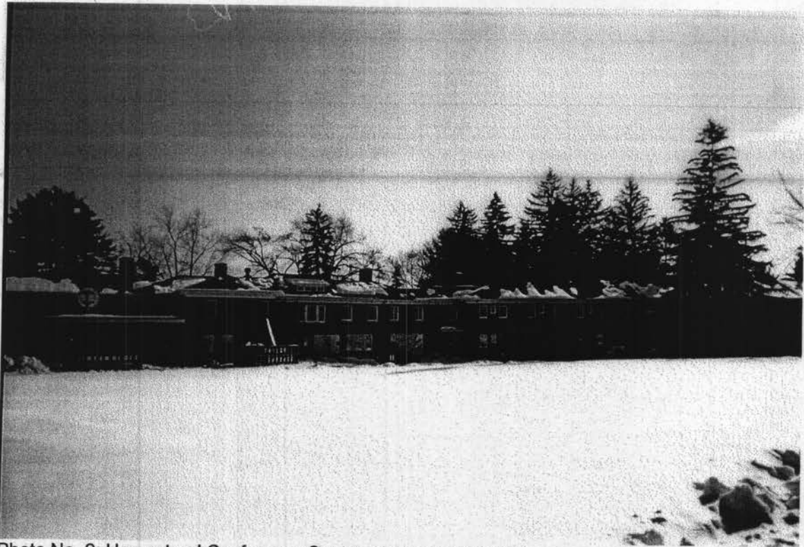
Photo No. 2: Homestead Conference Center, center and west end.
