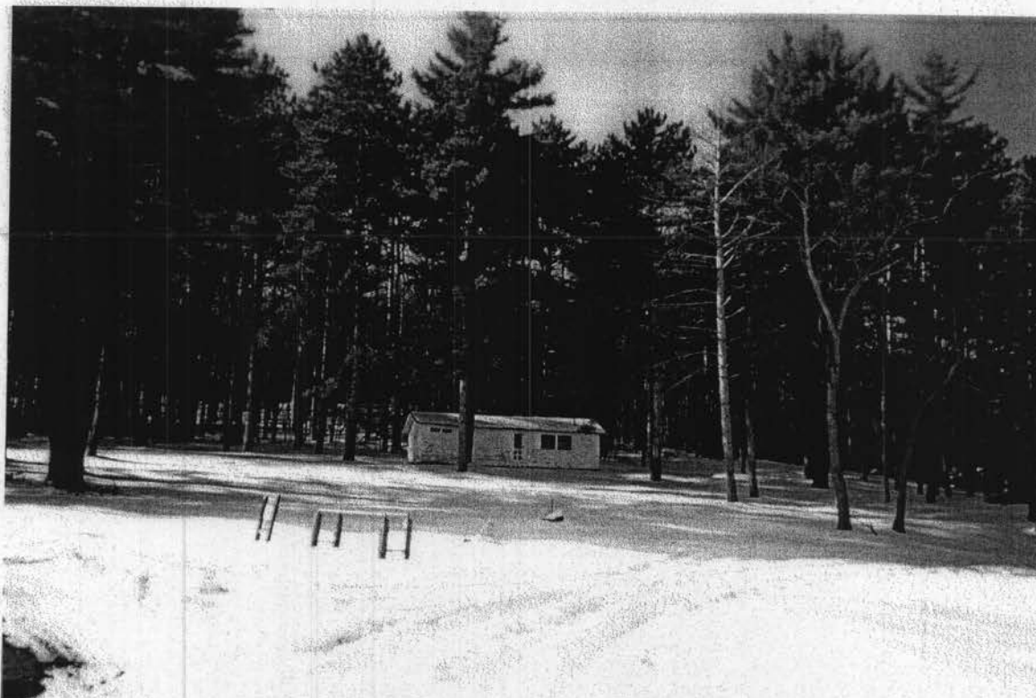
Photo No. 4: Small cottage-like building near Carriage House.
