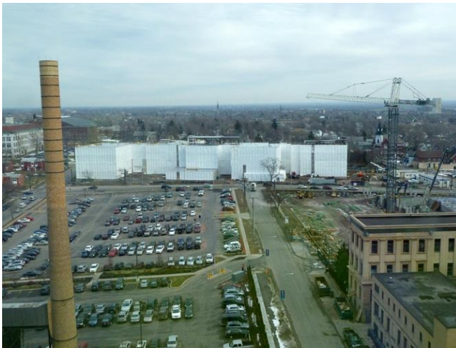
Facility under construction with panelized temporary shrouding
