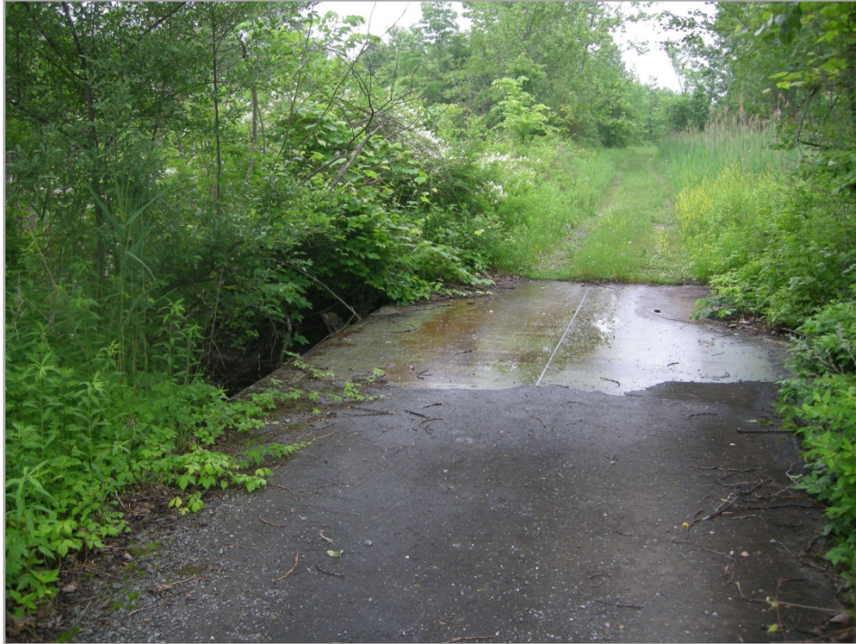
The Lot 65.22 portion of the site facing north.
