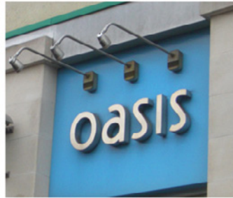
Contemporary cantilevered external illumination with cabinet construction sign below
