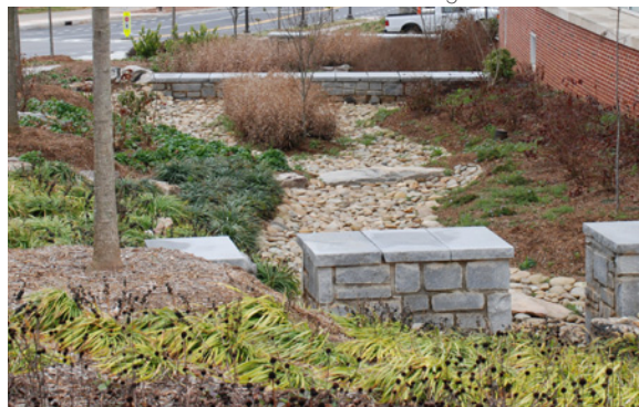
On-site rainwater infiltration recharges the local aquifer.
