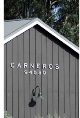
Wood cladding may be stained or painted, and may be detailed in a variety of ways. Both vertical and horizontal siding are permitted as well as louvered walls, rain screens, etc.
