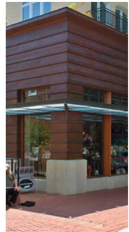
Metal cladding may be applied as siding, panels, rain screens, etc. Corten, copper, aluminum, perforated, corrugated, and brushed metals are permitted.
