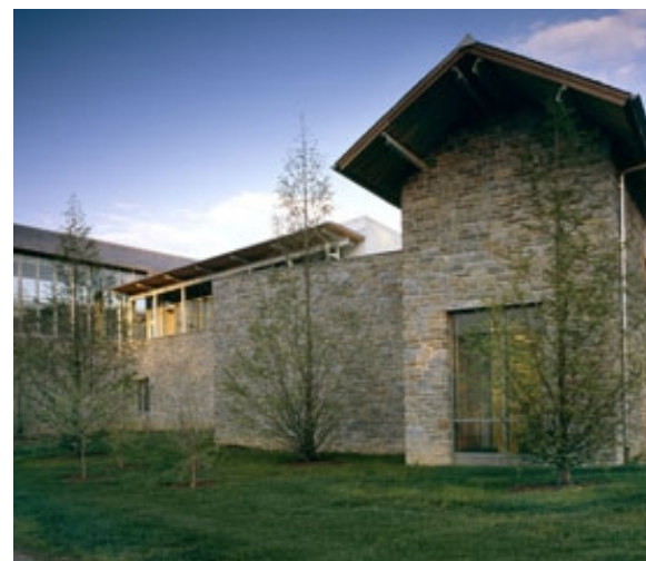
Where possible, a secondary façade should be broken up into smaller massing elements or use occasional glazing and material differentiation to avoid large blank surfaces.
