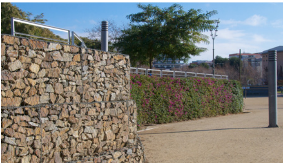
Site retaining walls are to be a maximum of 6'-0" and use materials that complement the associated architecture.
