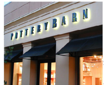
Halo illuminated fabricated letterforms attached directly to building fascia
