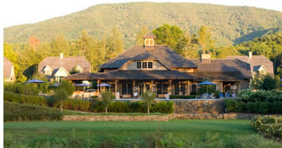
Hospitality buildings will reflect the legacy of Catskills hotels as offering a healthy environment - both indoors and outdoors - for visitors to enjoy.
