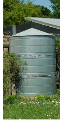
Use roof rainwater drainage for on-site irrigation or store in cisterns/rain barrels for future use.
