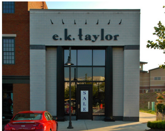
Window and door curtain wall systems should emphasize a building's vertical elements.
