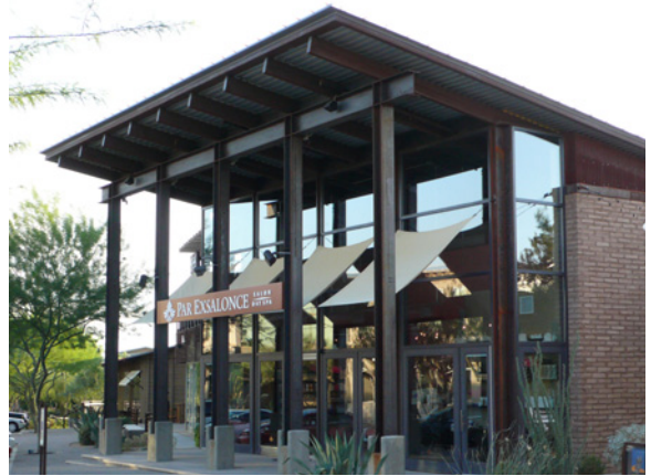
Overhangs that protect expanses of glass from excessive heat gain are encouraged.
