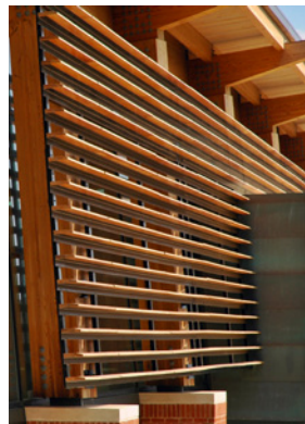
Wood cladding may be stained or painted, and may be detailed in a variety of ways. Both vertical and horizontal siding are permitted as well as louvered walls, rain screens, etc.
