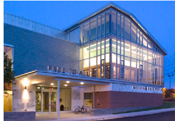
Double or triple-height glazing can be used to highlight a building's use.
