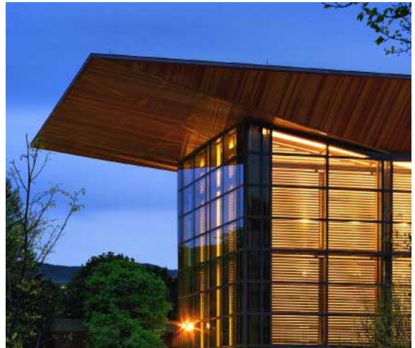
A broad sheltering roof can provide adequate protection from rain or snowfall while indicating a building's primary entrance.
