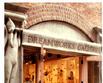
Carved and cast stonework at entry
