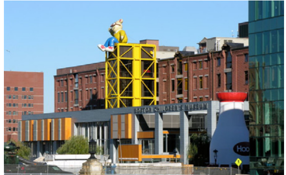
Civic/Institutional buildings geared toward a particular audience may consider using massing and unique features to attract residents and visitors.
