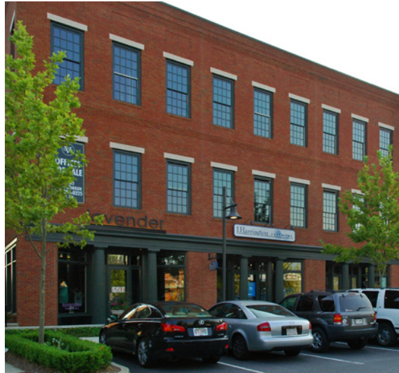
Punched windows and doors should use standard mullions; projecting head, jamb, and sill details; and projecting muntins.
