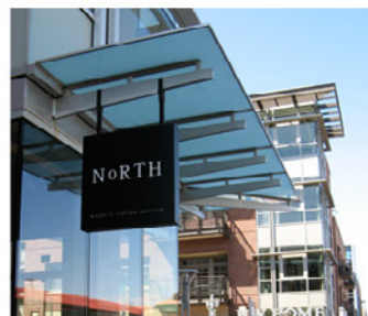
Clean thin profile cabinet construction arcade sign with minimal amount of backlit acrylic
