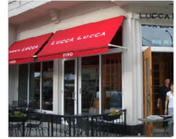
Fixed awning structure with graphics located on the primary (angled, typ.) surfaces
