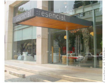
Canopy sign with graphics located on the sides of the structure
