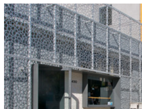
Metal cladding may be applied as siding, panels, rain screens, etc. Corten, copper, aluminum, perforated, corrugated, and brushed metals are permitted.
