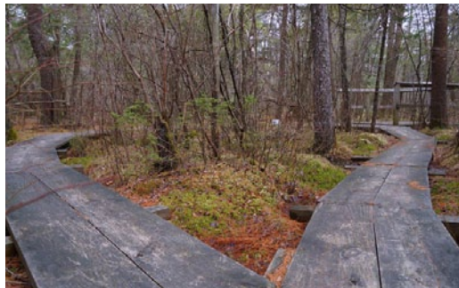
Boardwalk - Timber Plank
