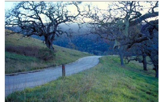
Finished roadway with trees preserved
