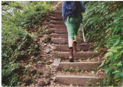
Wilderness Trail Timber Stair
