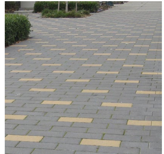
Asphalt Paver at Trail/ Road Intersection (Color contrast)
