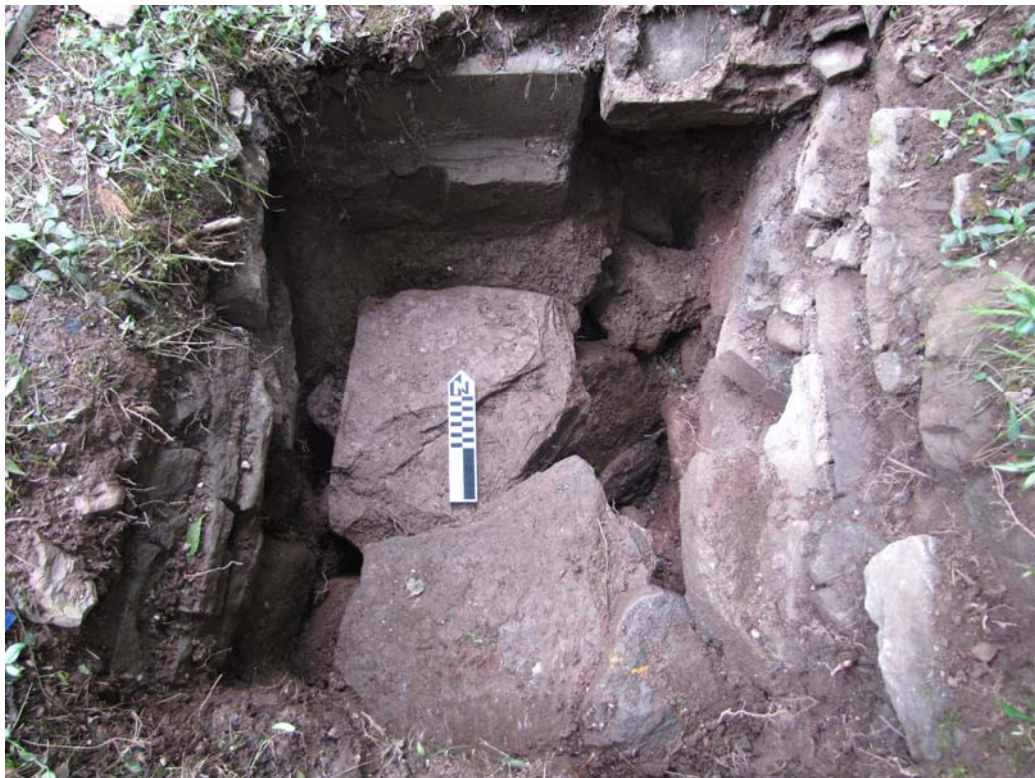
Photo 33: View of Unit 6 showing foundation to left and top with additional stone retaining wall at right.
