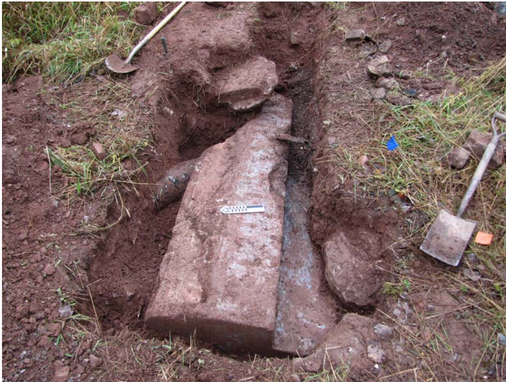
Photo 54: View east across expanded Unit 7 showing concrete steps encountered below ground surface.
