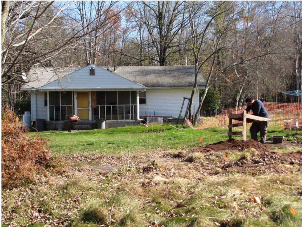
Photo 52: View east showing excavation of Unit 6 at end of concrete sidewalk.
