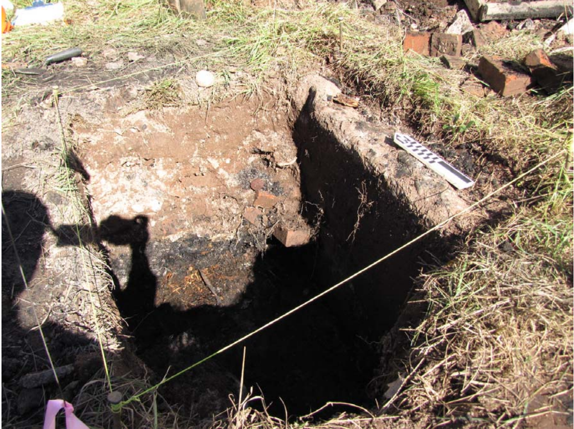
Photo 48: View northeast of Unit 3 showing concrete foundation and mass of rusted nails on floor.
