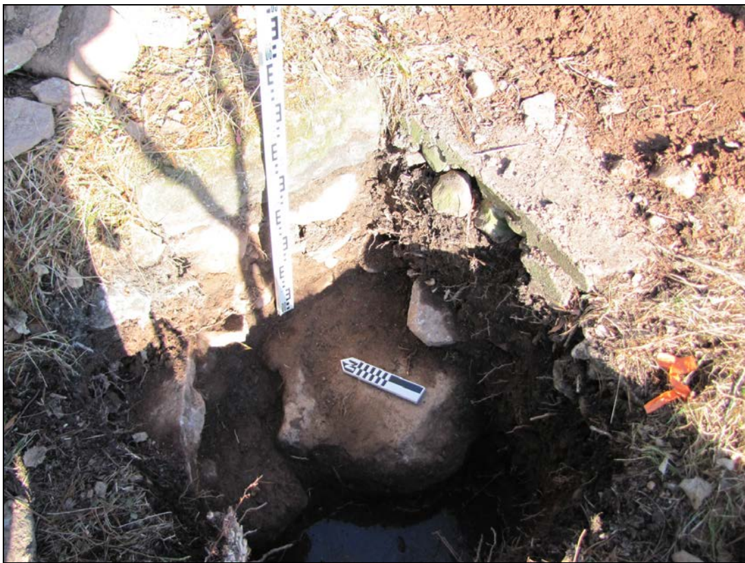
Photo 41: View northeast of Unit 3 with foundation at left, concrete sidewalk at right.
