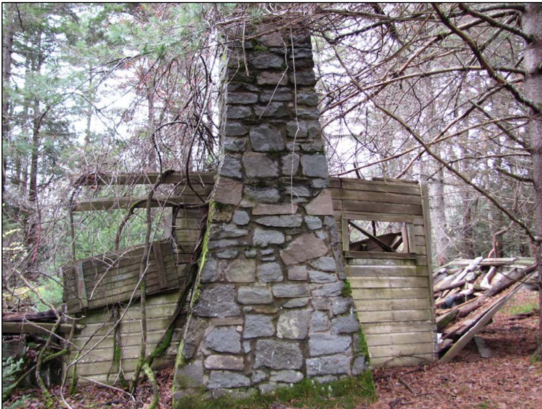
Photo 10: View west toward cottage remains showing exterior of stone fireplace.
