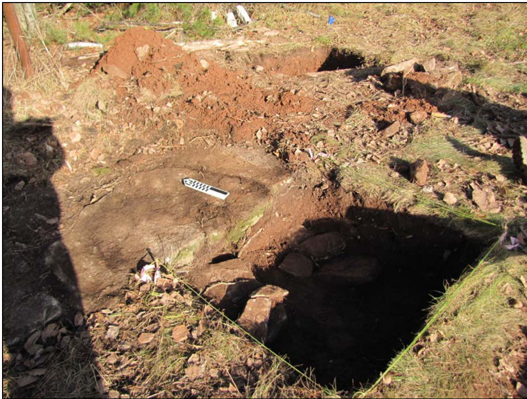
Photo 45: View northeast of Unit 21 at front edge of concrete platform with Unit 17 at rear.
