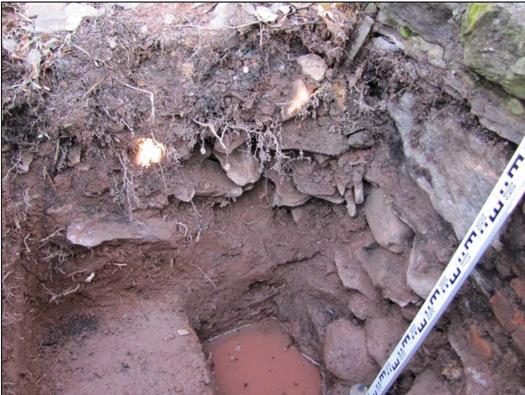
Photo 34: View north of Unit 1 showing loosely stacked stone in upper strata adjacent to foundation.
