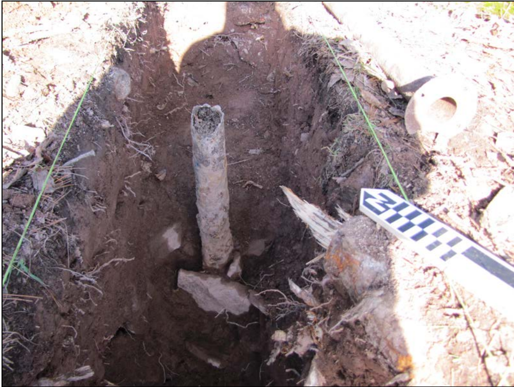
Photo 49: View north of broken porch support base showing thin stones packed around bottom.
