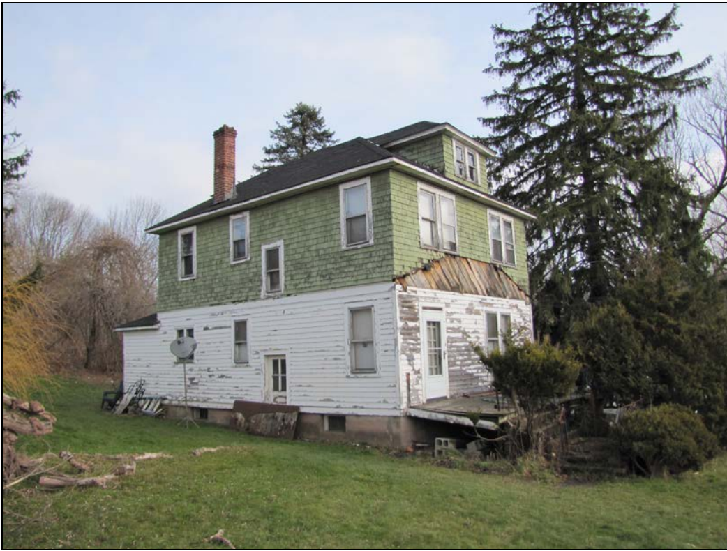
Photo 6: View northeast of residential structure on Cimarron Road.
