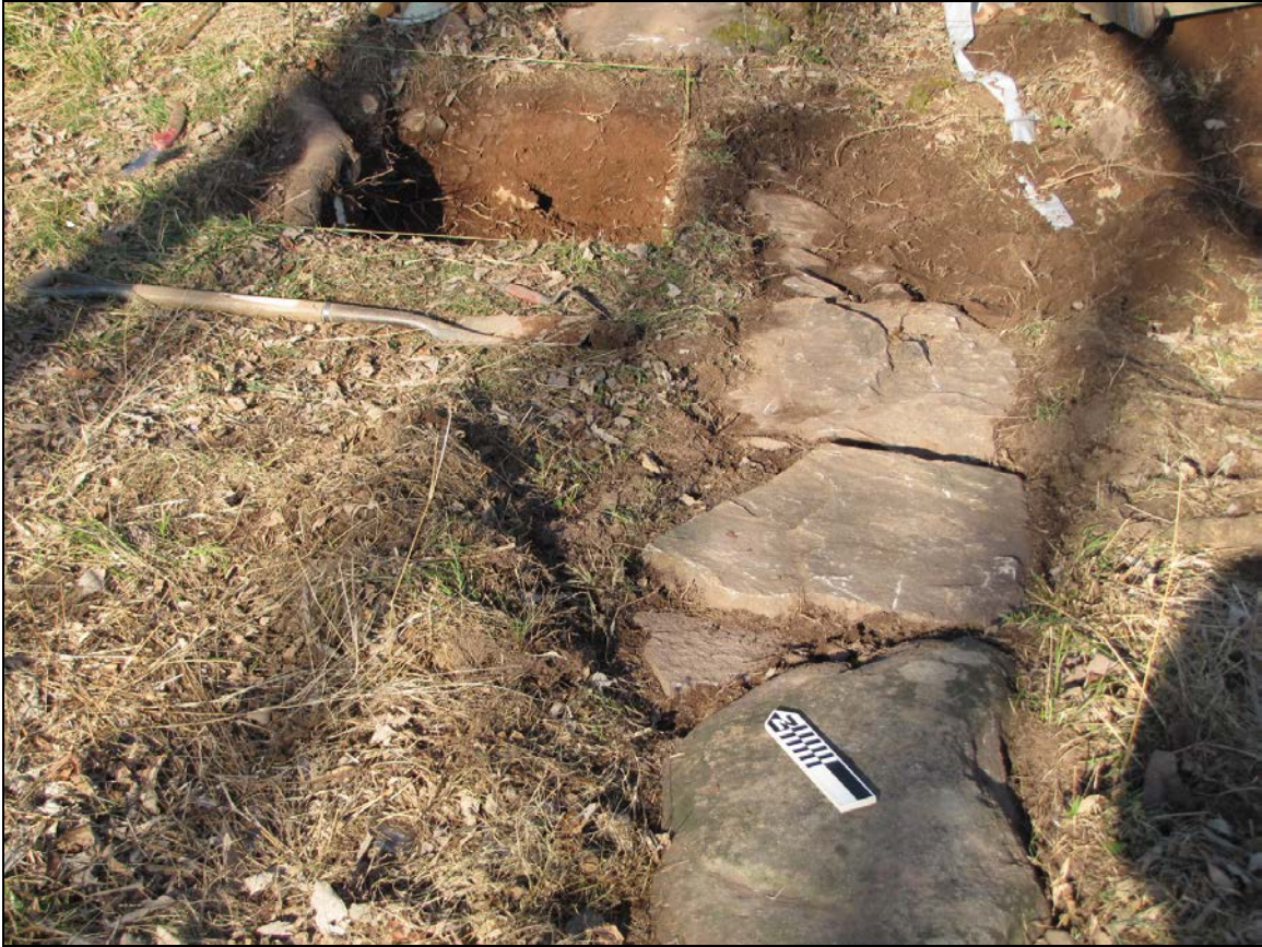
Photo 16: View northeast of foundation wall and Unit 7 excavation inside northeast corner of foundation.
