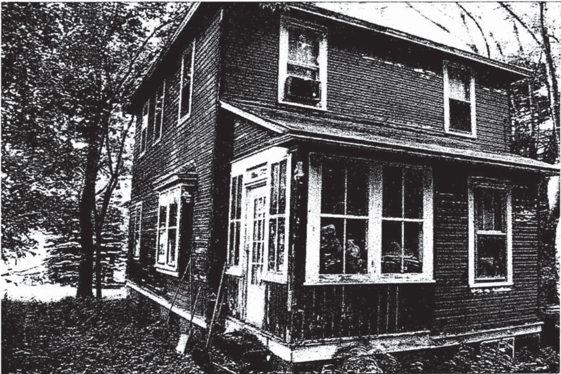
Rear and east elevations, facing southwest.
