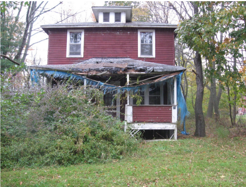
View of the south (Cimarron Road) façade.
