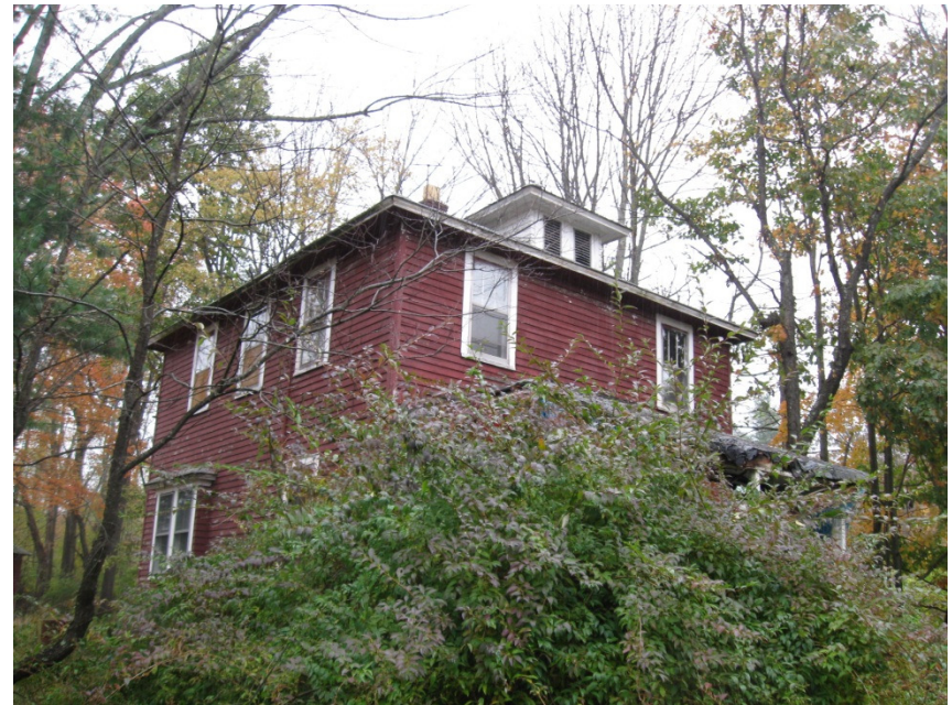
View northeast, including the west façade.
