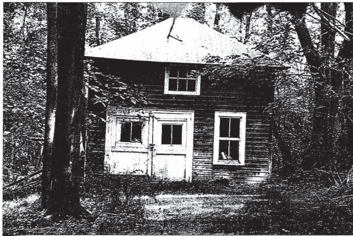
South elevation of the garage, facing northwest.
