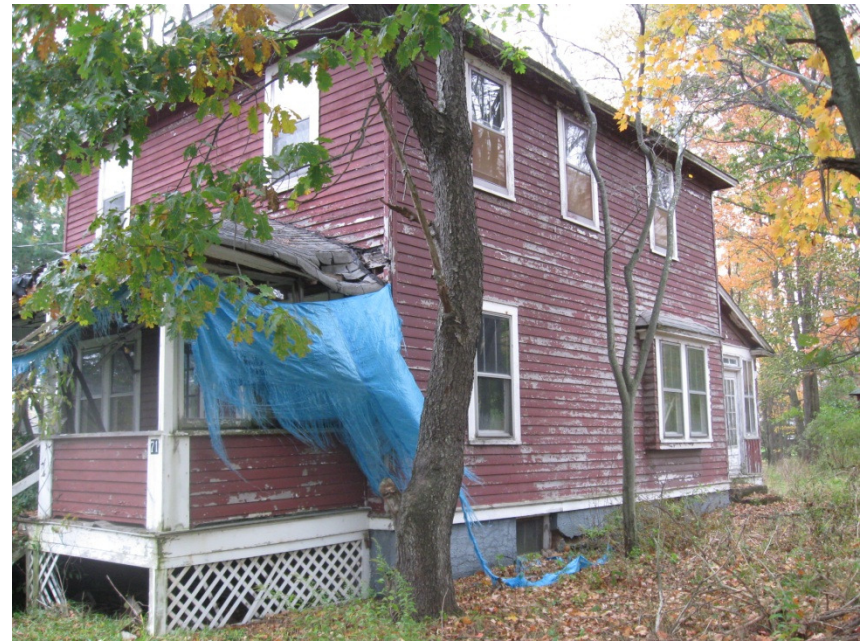
View northwest, including the east façade.
