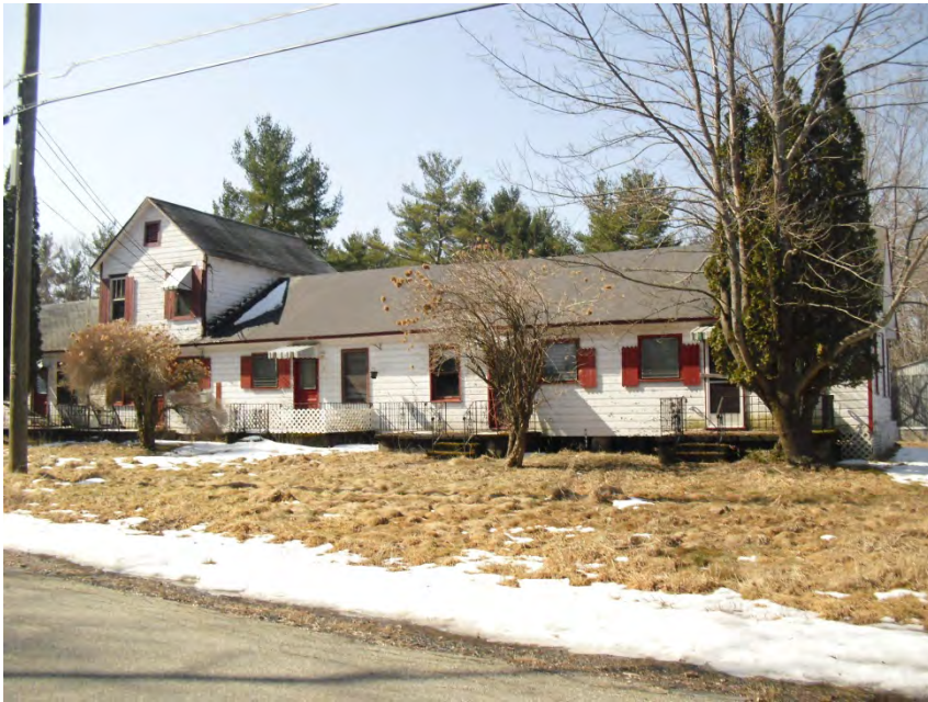
Central bungalow/office building, view southwest from Joyland Road.
