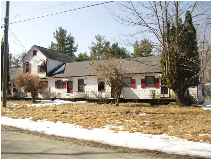
9. Central bungalow/office building, view southwest from Joyland Road.
