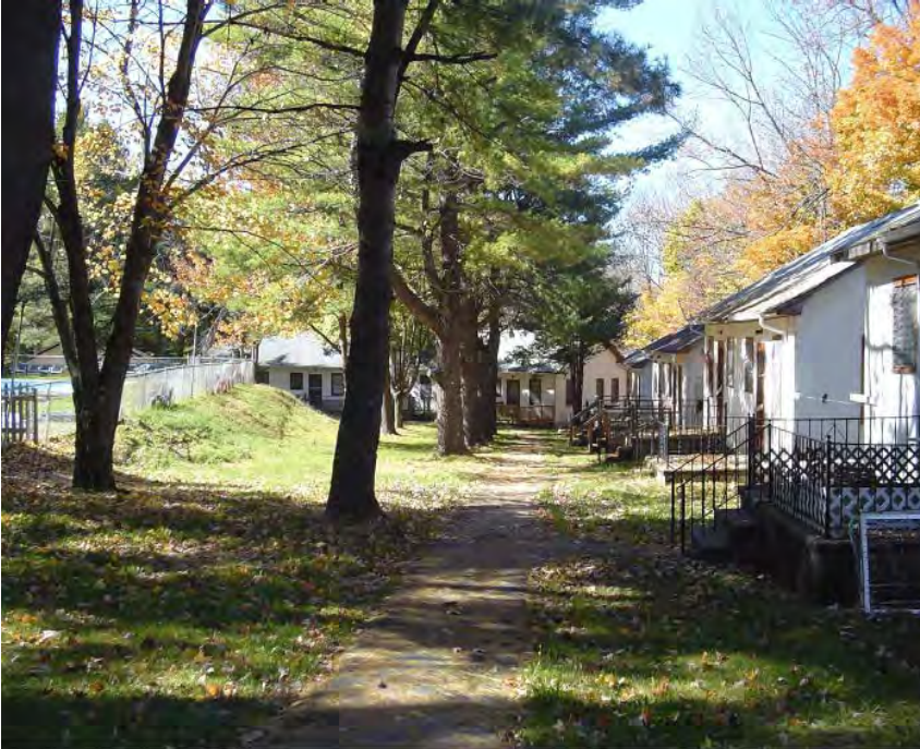
Breezy Corners bungalows, north grouping, view northwest of the pool facades of the bungalows. The pool is on the left.
