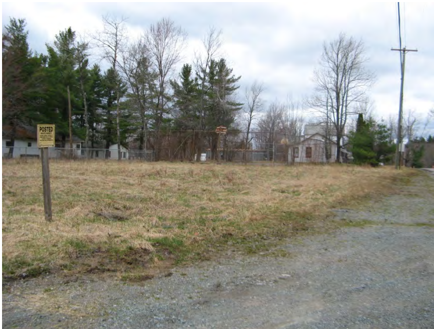
13. View north of the south façade of the central bungalow/office building , the basketball court, and cottages to the west.
