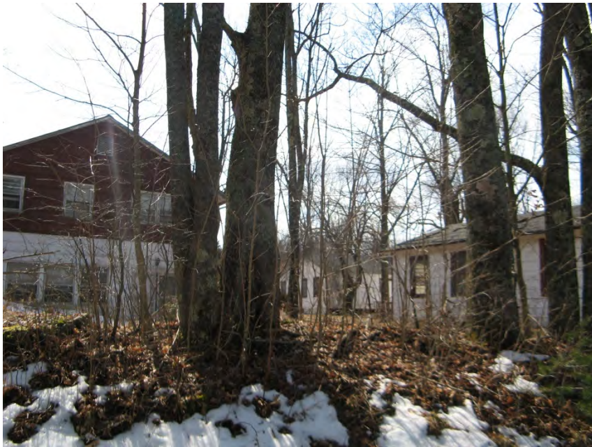
5. View south from Thompsonville Road of ranch house at corner of Joyland Road and bungalow building to the west.
