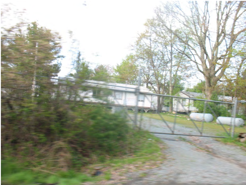
View north from Towner Road of bungalows.
