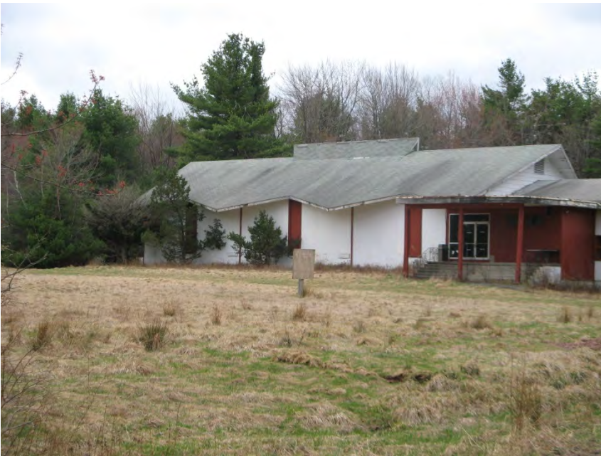
19. South end of the Casino/Recreation Hall.
