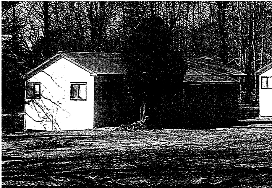
Photo 4. View northwest of structure 3.
