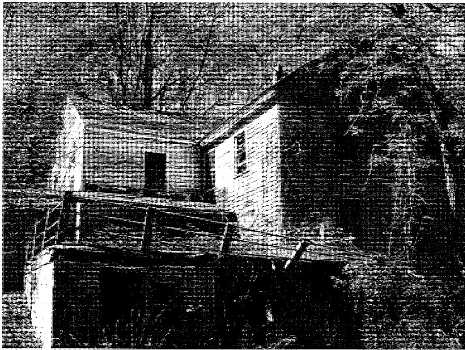
Photo 2. View of 374 Thompsonville Road looking west.
