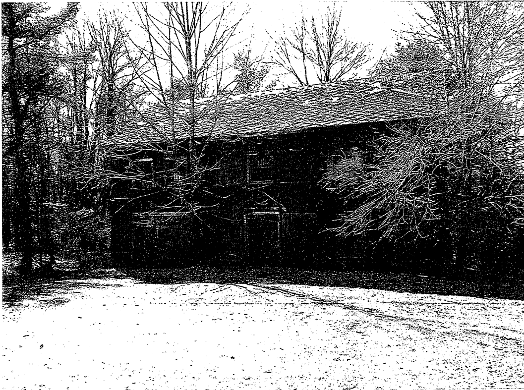
Photo 4. View west of the barn associated with the J. Gray house.
