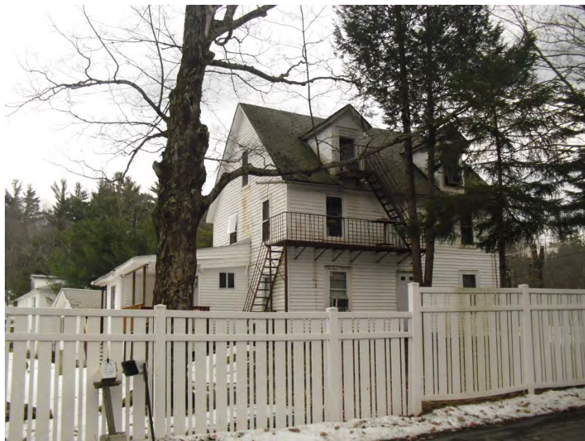
View east from Joyland Road at house at 130 Joyland Road.
