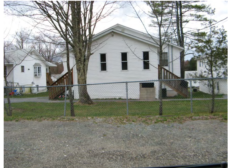
View west from Joyland Road of one of the two-story Bungalow Colony buildings.
