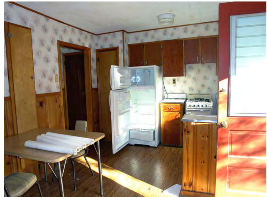
Representative kitchen in the central bungalow/office building. Source: www.vanishingcatskills.us
