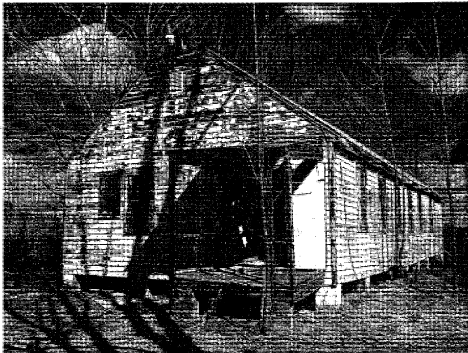
Photo 5. Recreation pavilion looking northeast. This building was razed in 2006.
