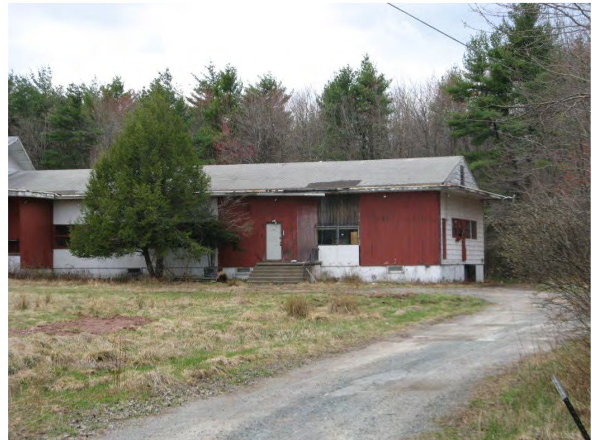
20. North end of Casino/Recreation Hall.
