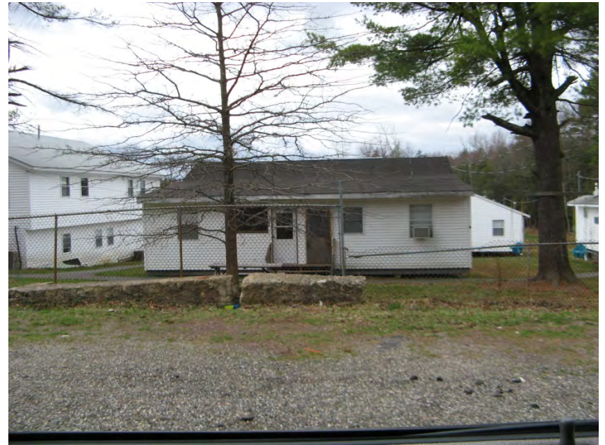
View west from Joyland Road of northern Bungalow Colony buildings.
