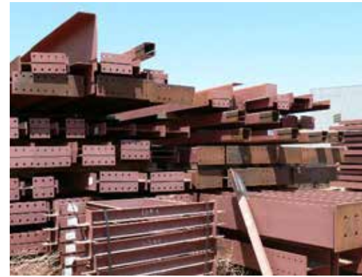
All Steel is Fabricated and Ready for Delivery
