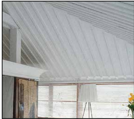
[ wood batten ceiling ]
