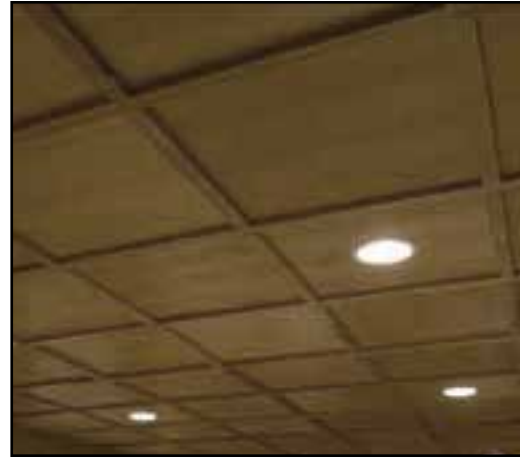
[ coffered lay-in ceiling ]
