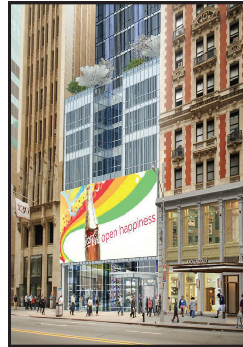
New hotel in Times Square (under construction)
