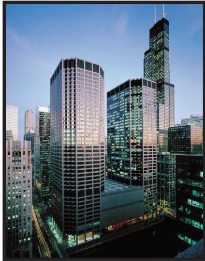
Chicago Mercantile Exchange Center, Chicago, IL
