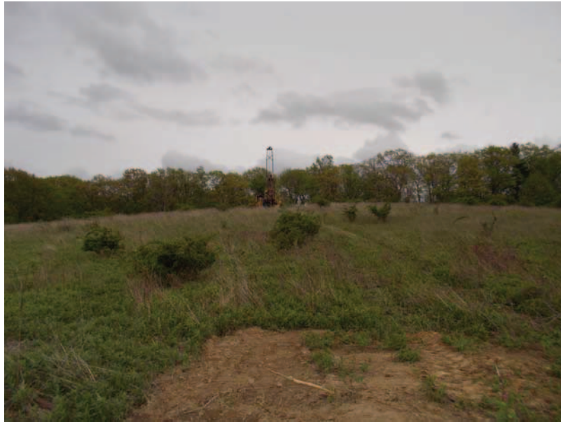
Drilling B-1, looking east Note: Variable surface topography
