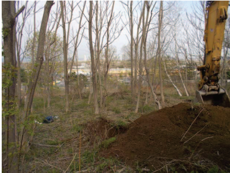
Advancing TP-1, looking west
